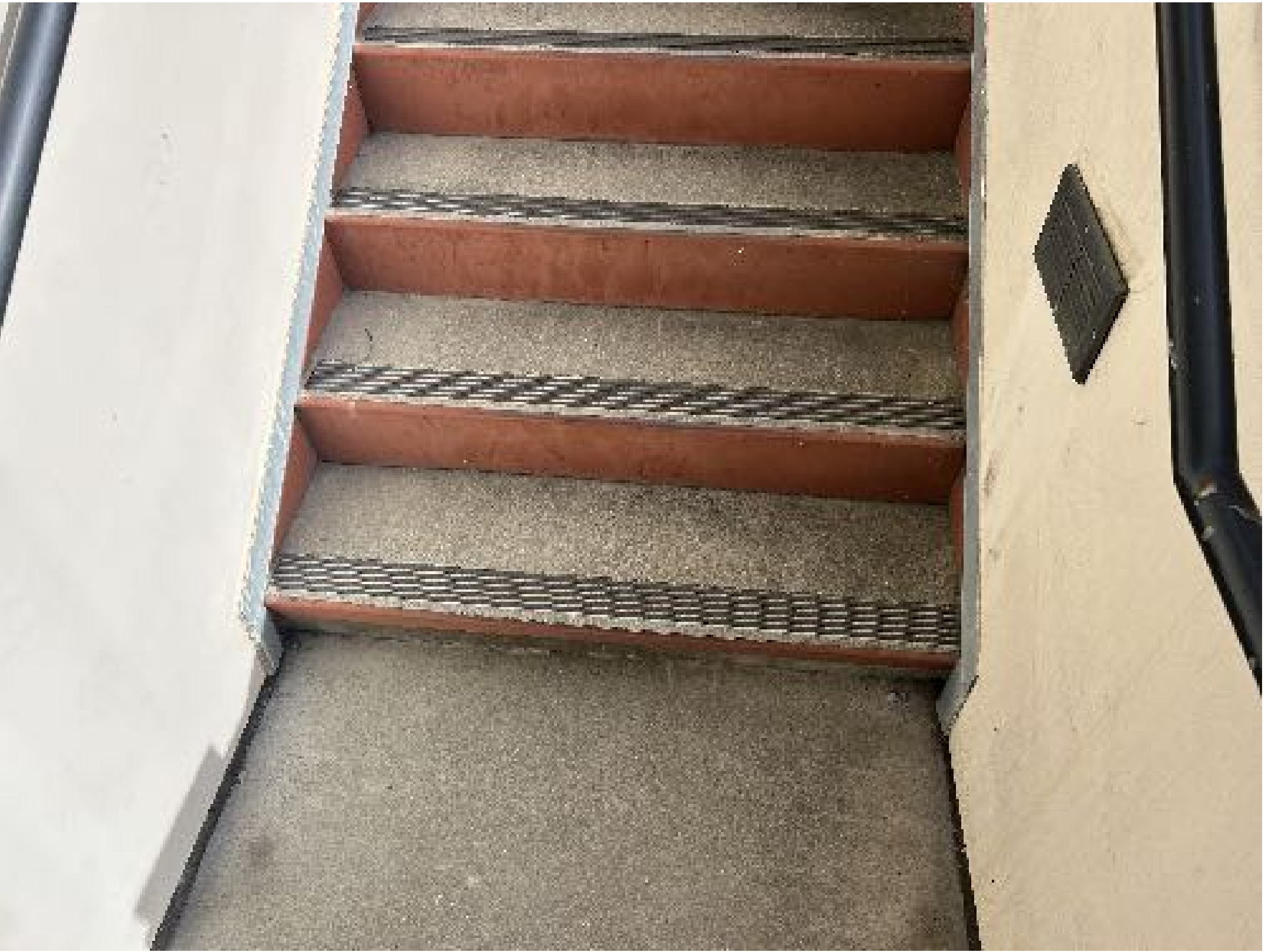
EXISTING STAIR CONDITIONS
