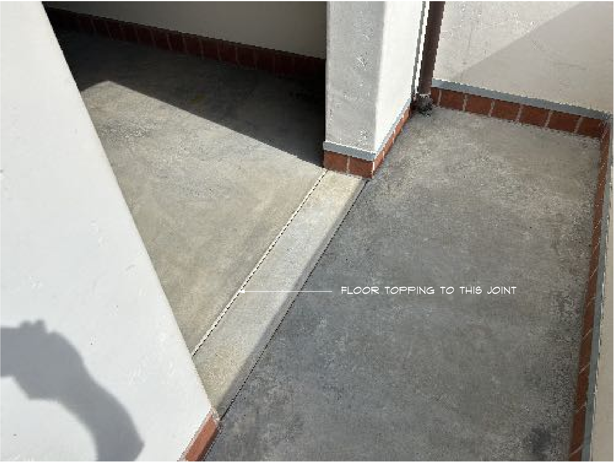
EXISTING FLOOR FINISHES
