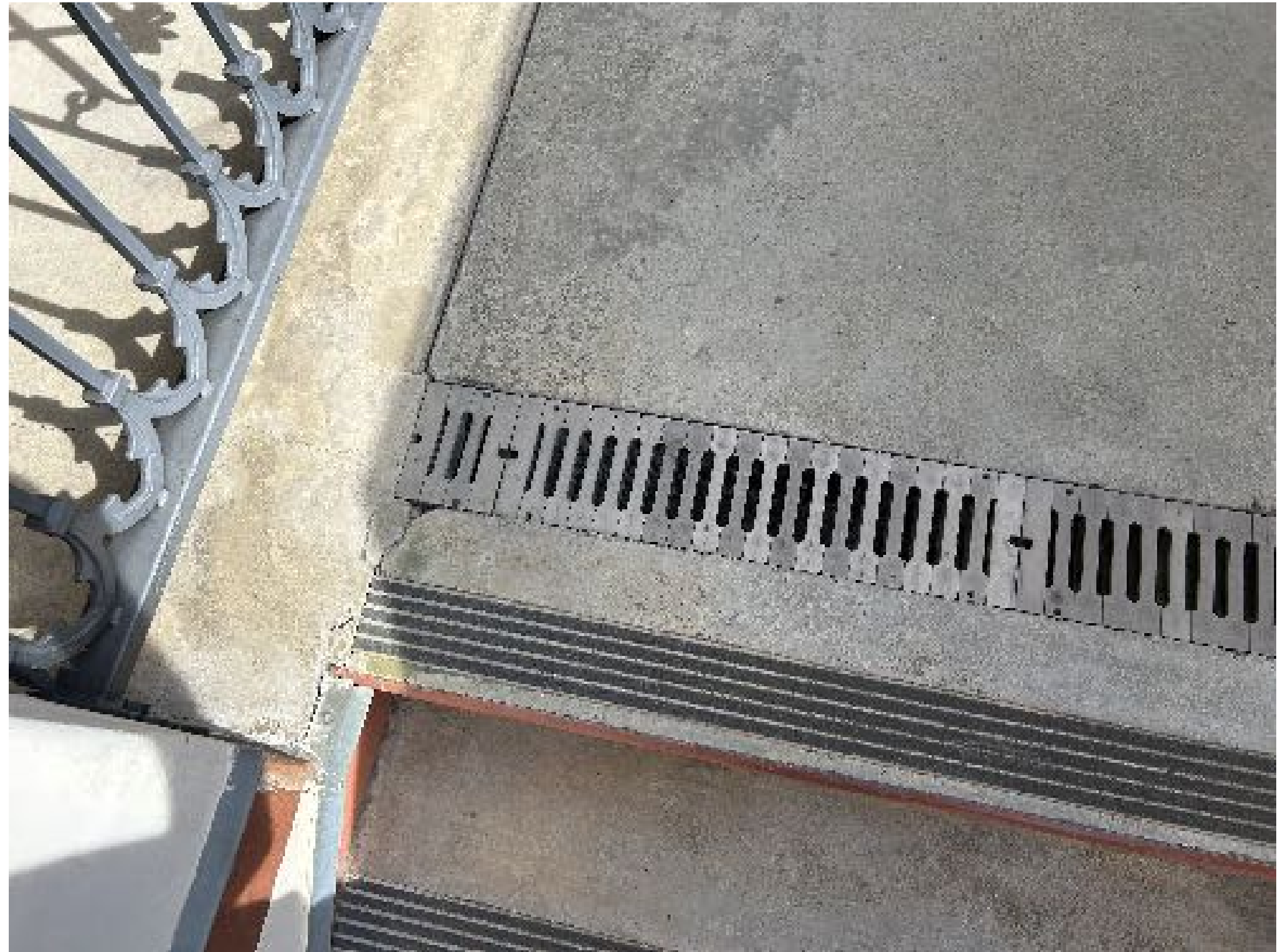
TOP OF STAIRS/EXISTING TRENCH DRAIN
