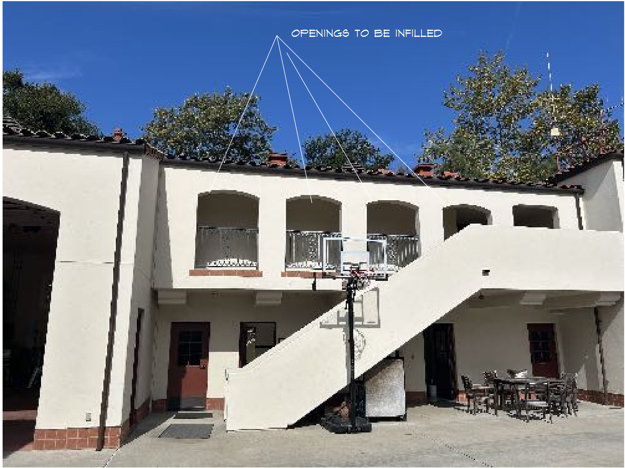
OVERALL VIEW OF STAIRS/OPENINGS TO BE INFILLED
